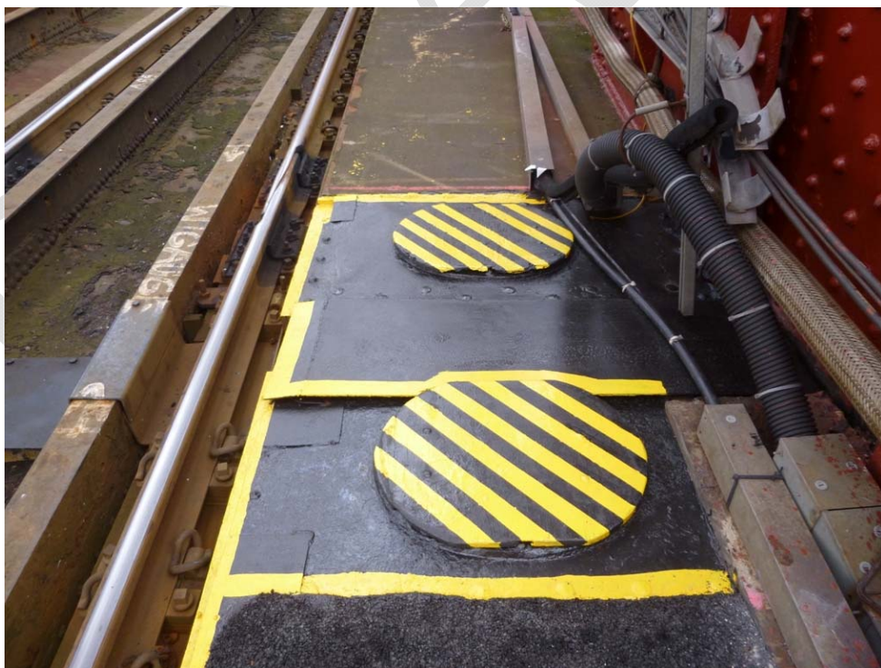
Cess walkway exposed steel and timber lids after preparation and coatings
