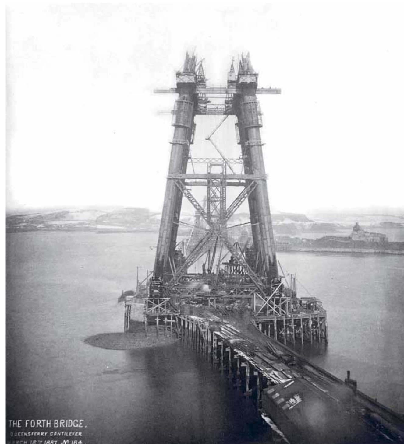
Photograph showing progress of the Queensferry main tower on 12 March 1887, (© Crown Copyright, National Records of Scotland).
