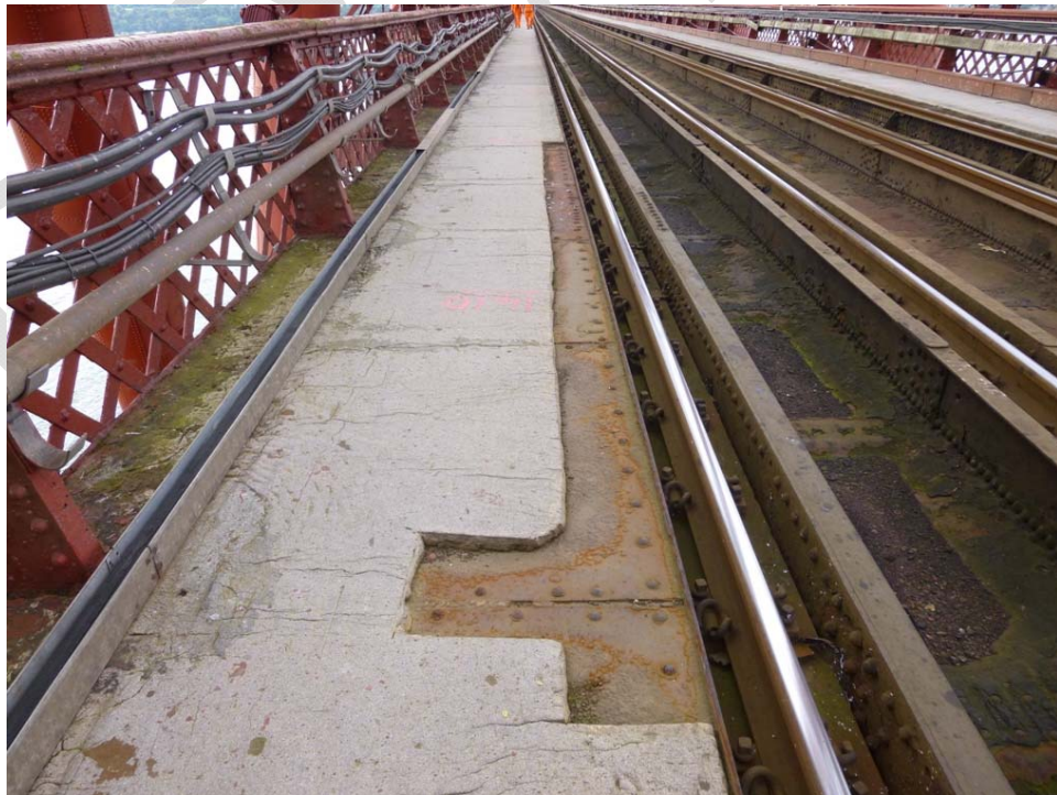
Typical condition of cess walkway
